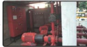
FIRE PUMP HOUSE
